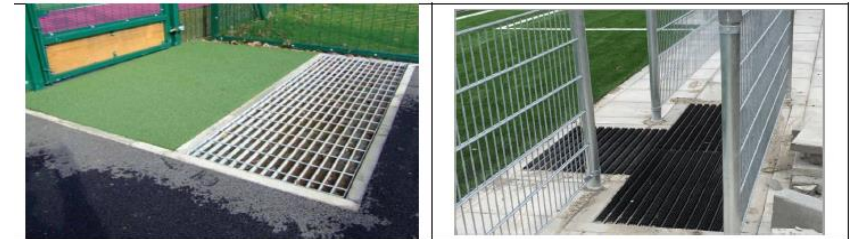
Catchment gates and grids at pitch entrances 18,19
